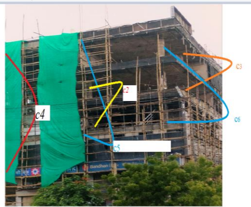
Figure 3 External View of Post Fire Building
