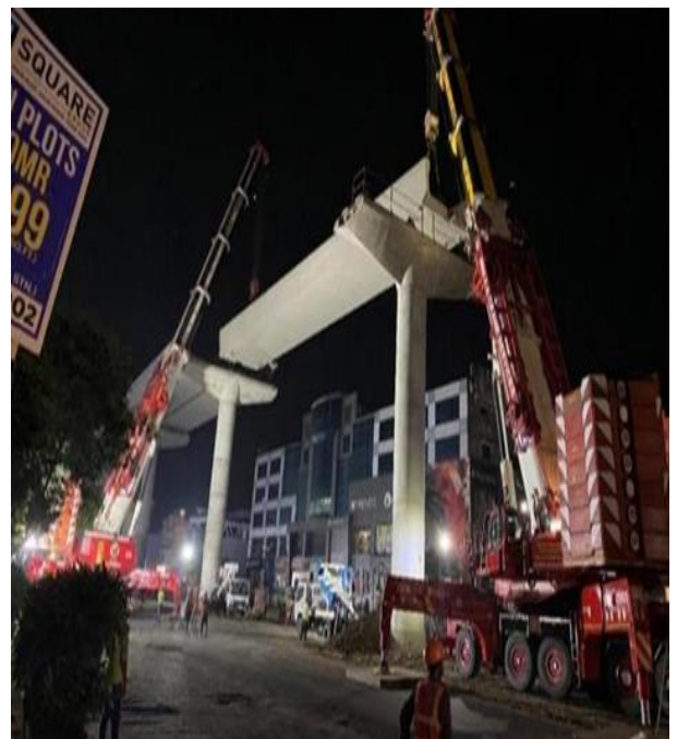
Figure 3 Process of U Girder Erection
