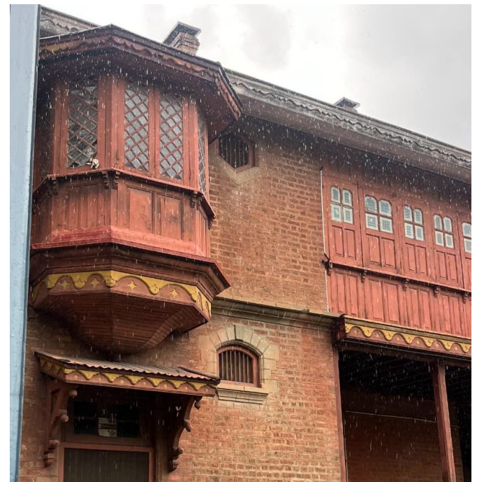
Figure 8 Intricately Ornamented Jharokha-Style Bay Window
