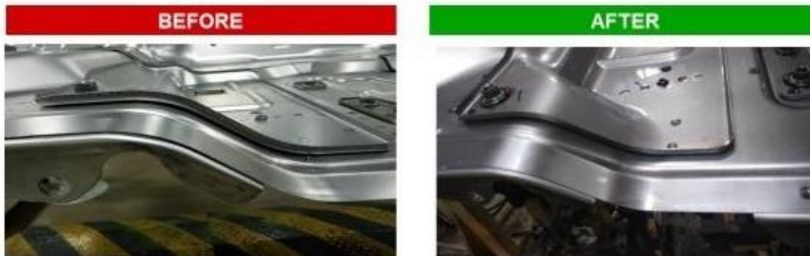
Fig.4.Effect of defect in Seat Mounting gap in L61095
